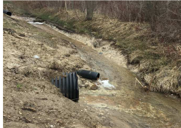
Photograph 2: Culvert and tile drainage out-sources at point of confluence (~200m upstream of property boundary)
