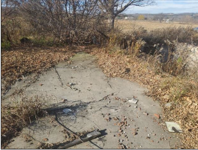
Image 3: View of a concrete surface associated with the former farmhouse within the west portion of the former farm complex.
