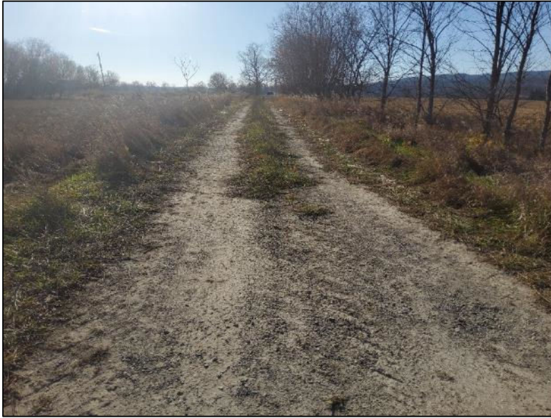
Image 1: View of the compacted gravel driveway providing access from Edward Street East to the former farm complex.
