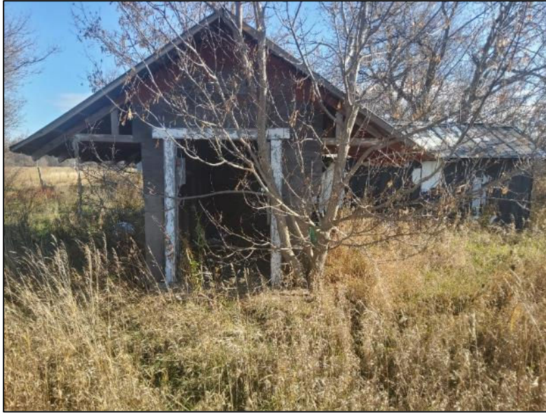
Image 5: View of an animal shed within the former farm complex.
