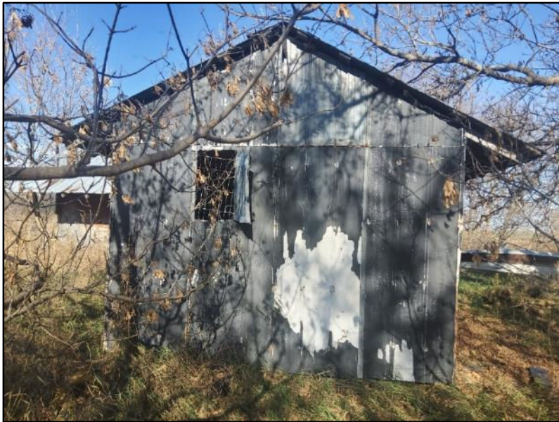
Image 6: View of a storage shed within the former farm complex.
