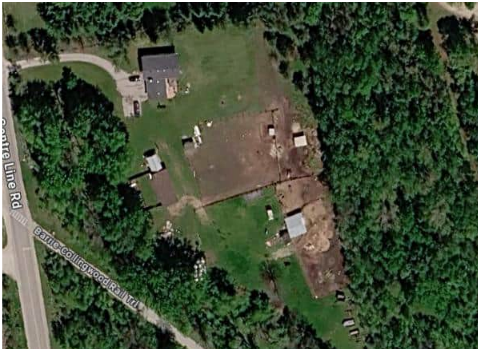
29 Aerial 1415 CENTRE LINE RD
