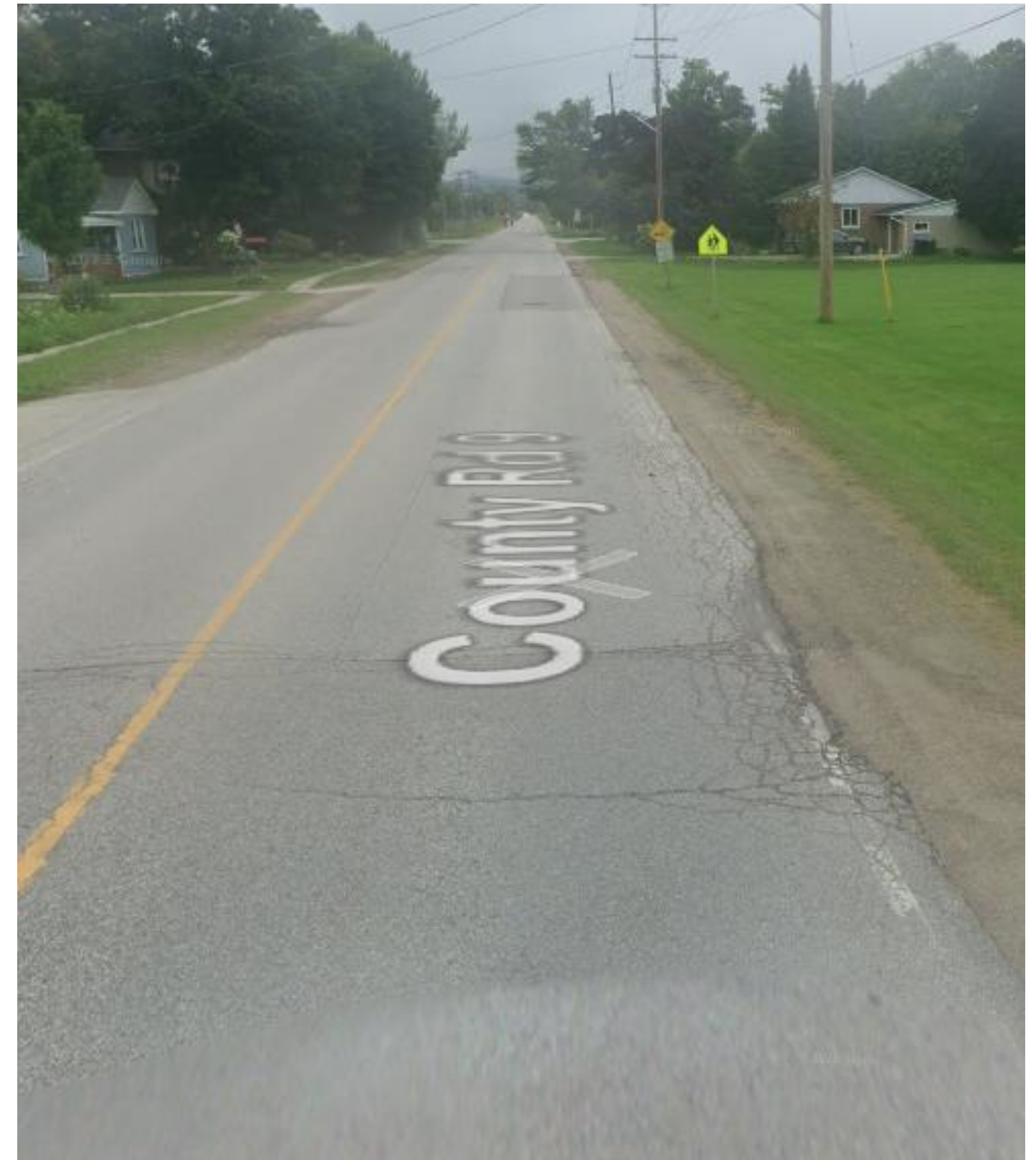
Looking west along County Road 9 from access
