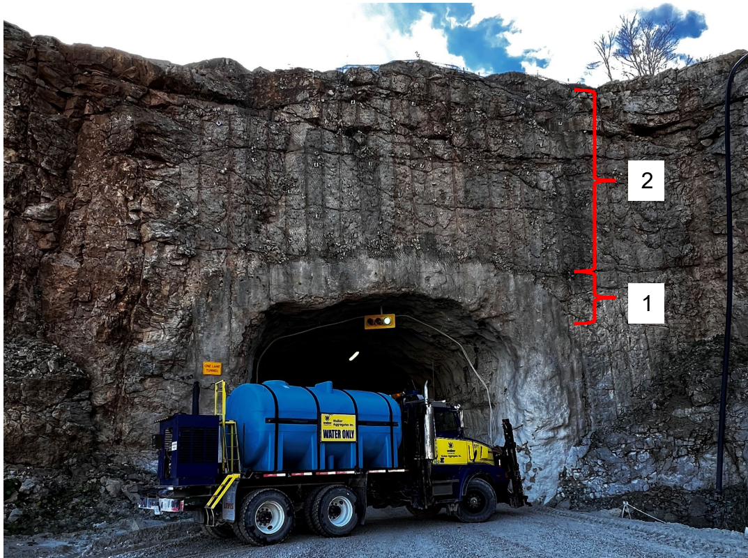
Area around the tunnel opening supported with reinforced shotcrete and rock bolts (1). Upper rockface area (2) supported with wire mesh and rock bolts. Areas along the portal with cracked and loose shotcrete, some areas with shotcrete missing. No seepage/moisture noted at the rockface.
