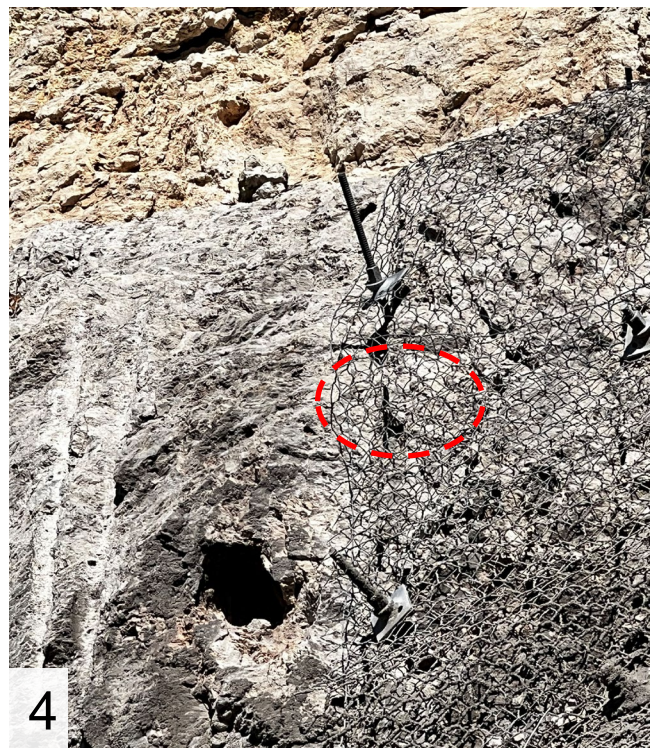
Rock bolt plate not tight to mesh on the west side
