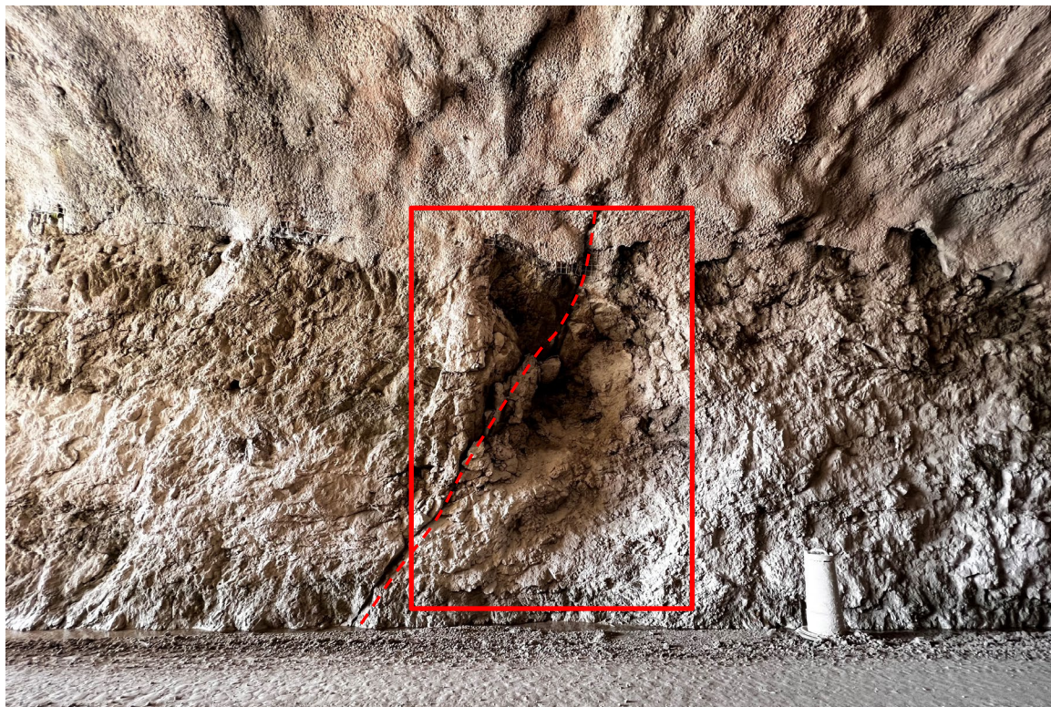
Chainage 0+23 m. Weathered area with open discontinuity (dashed line) and small to medium sized loose blocks (see left below) and a large unsupported block with potential to fall (on right below)
