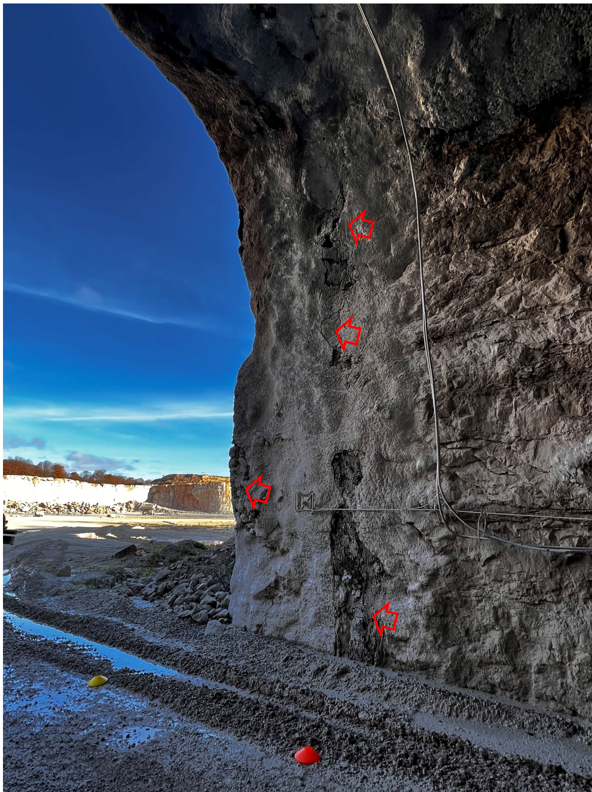
Shotcrete cracking and areas with exposed rock observed near the north portal.
