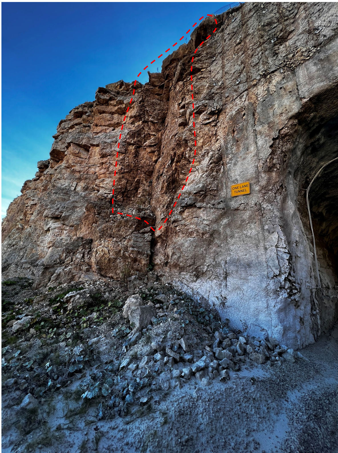
East face adjacent to north tunnel portal: Weathered rock mass with loose blocks and large overhang supported with rock bolts at slope crest. Rock debris accumulated along the rock face toe at tunnel entrance.
