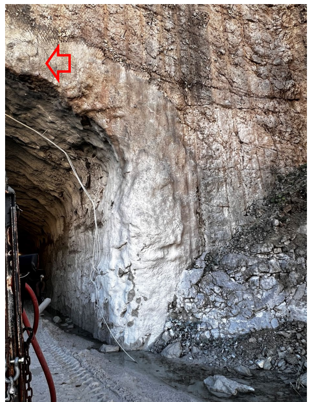
West: Minor cracking in shotcrete on lateral edges of the north portal face.
