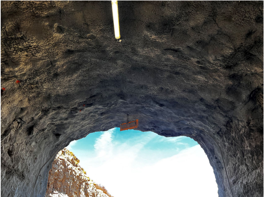
Overview of crown near North Portal. Shotcrete in good condition in the crown. Areas of hollow and cracked shotcrete smaller areas with exposed wire mesh and rock mass (in red below ).
