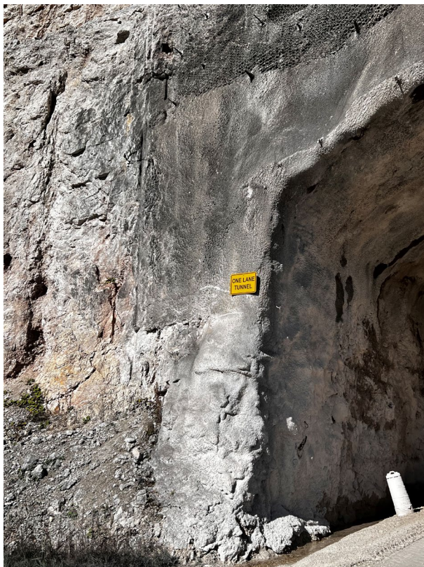
West: Shotcrete on lateral edges of the south portal face in good condition.
