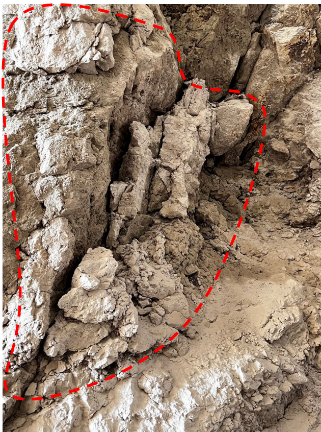
Chainage 0+23 m. Weathered area with open discontinuity (dashed line) and small to medium sized loose blocks (see left below) and a large unsupported block with potential to fall (on right below)
