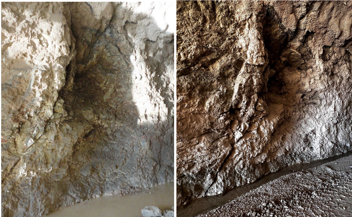
Figure 1: Weathered rock mass at chainage 0+23 m, photograph taken in 2015 (left) and photograph taken in 2023 (right).
