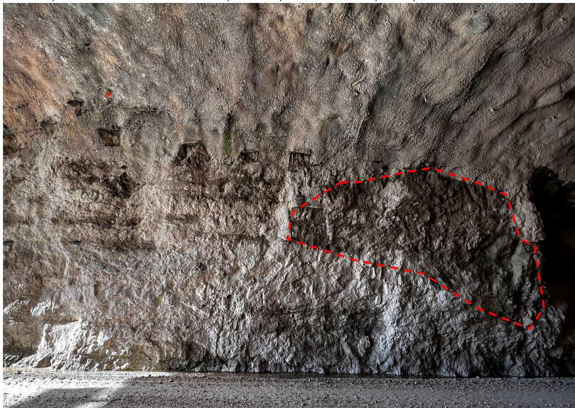
0+10 to 0+20 m. Shotcrete generally very thin in haunches. Some dampness noted along the tunnel haunches near where the water is drained by the drainage panels.
