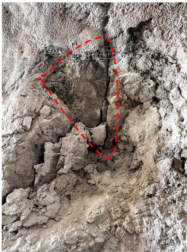
Chainage 0+23 m. Weathered area with open discontinuity (dashed line) and small to medium sized loose blocks (see left below) and a large unsupported block with potential to fall (on right below)
