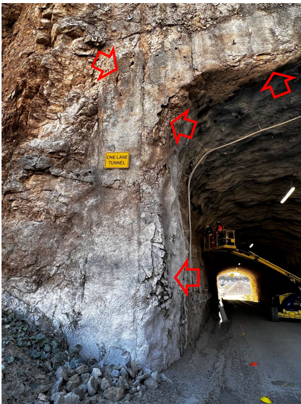
East: Areas with loose shotcrete and cracking in shotcrete and exposed rock on lateral edges of the north portal face.
