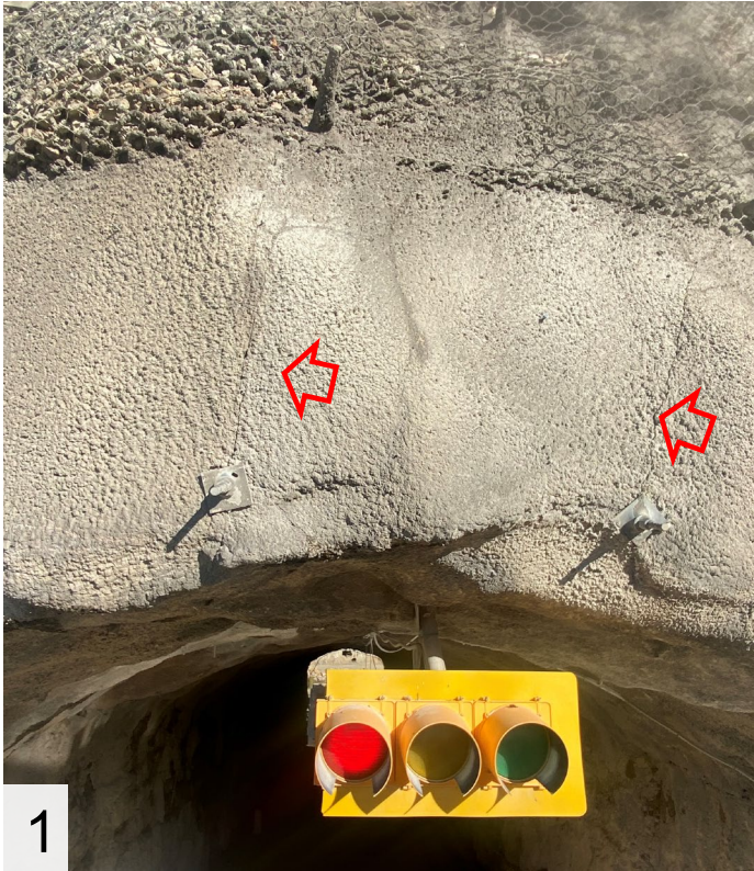
Two vertical cracks (1-2mm wide) in shotcrete above the portal..
