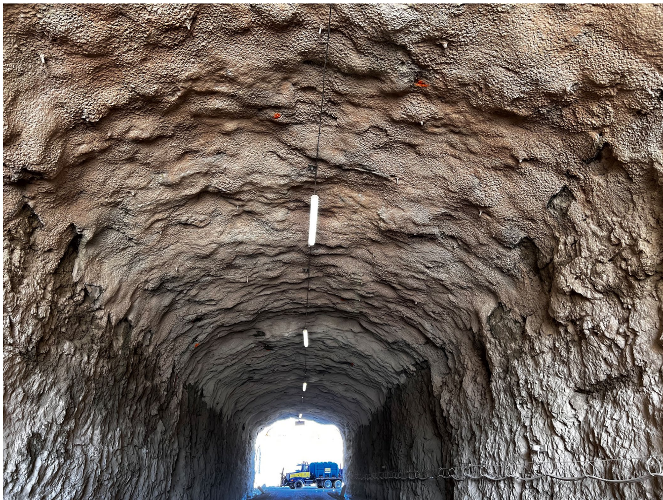
Overview of shotcrete condition in the crown at chainage 0+45 m toward the North Portal. Dry conditions with some hollow areas.
