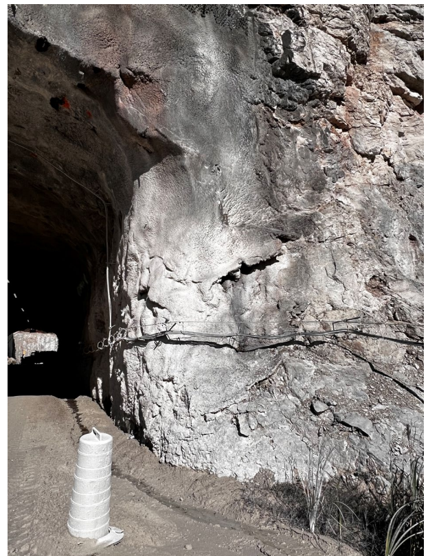
East: Shotcrete on lateral edges of the south portal face in good condition.
