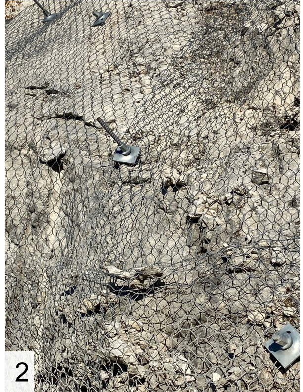
Rock debris accumulated behind the mesh.
