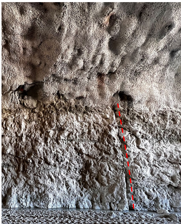
Left: Small loose blocks along the vertical discontinuity (dashed line) at 0+69 m.
