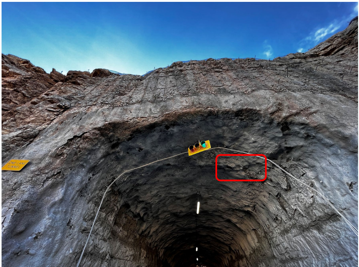
Overview of crown near North Portal. Shotcrete in good condition in the crown. Areas of hollow and cracked shotcrete smaller areas with exposed wire mesh and rock mass (in red below ).
