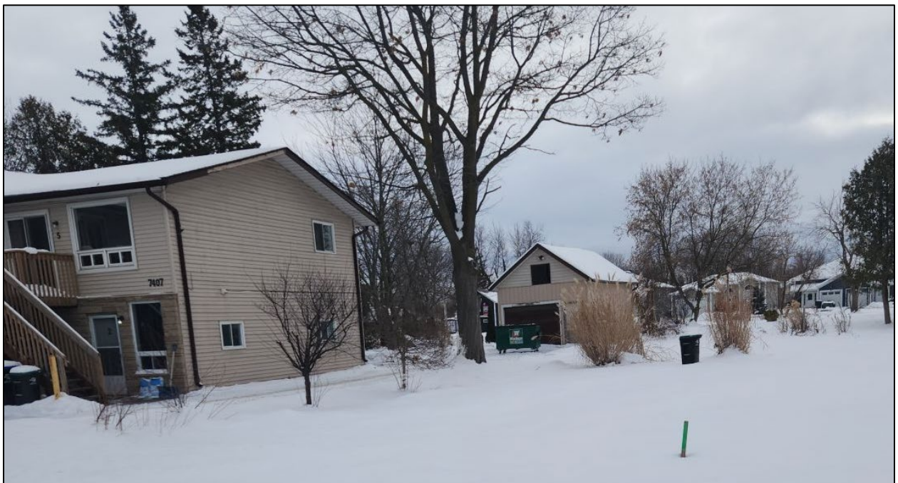
Figure 6: Existing Six-Plex and Accessory Structure on the Subject Lands (Facing South)
