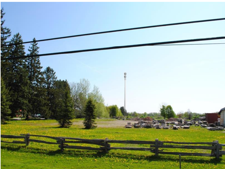
View from County Road 124, looking east towards the tower location, at an approximate distance of 0.45km from the structure.
