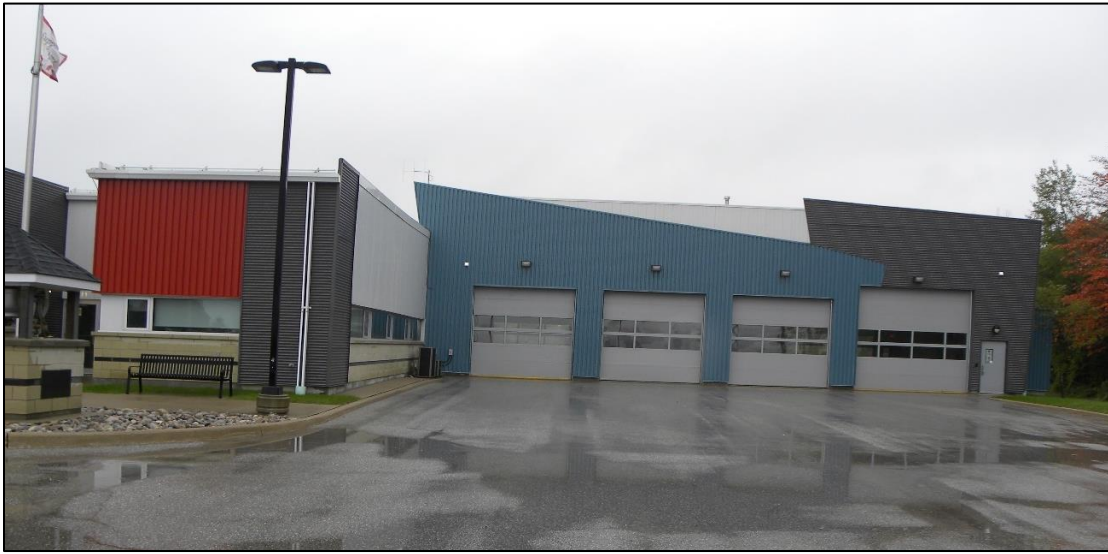
Front Entrance (also serves as a Safe Room)
